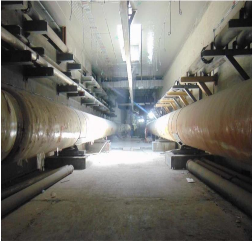
SUB- CHILLER LINES WORKS
