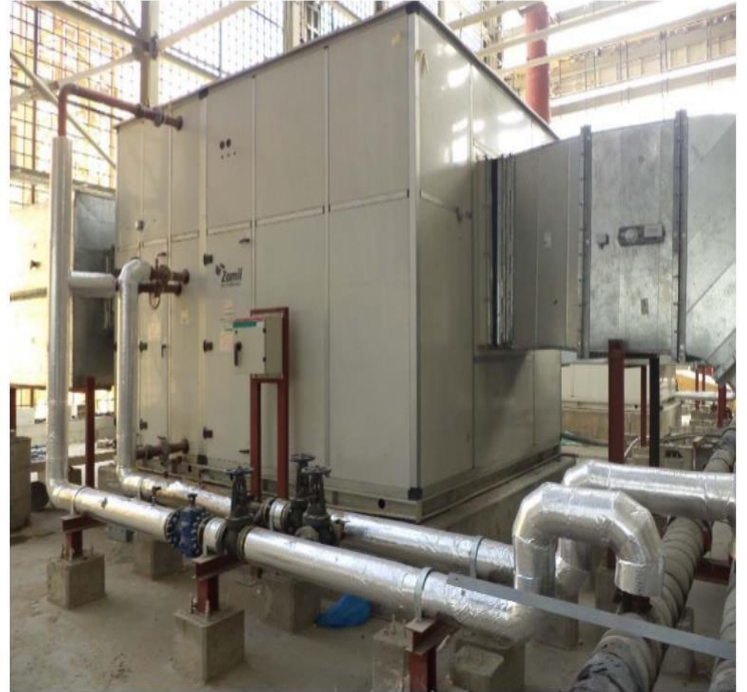
CHILLER SYSTEMS MECHANICAL WORKS
