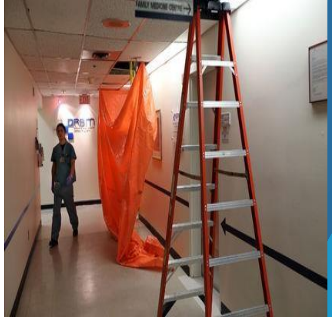
HVAC INDOORS MAINTENANCE
