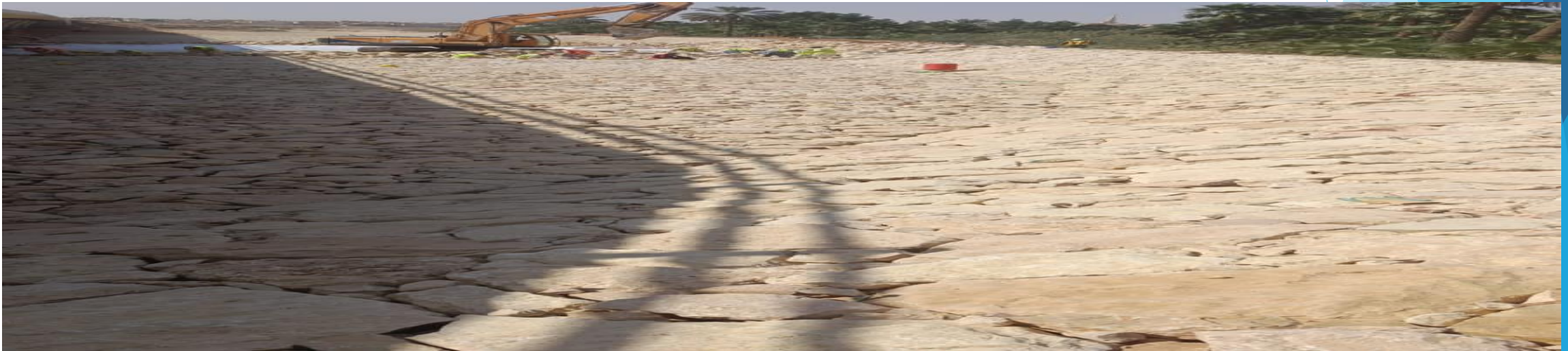
RIP ARAP AND GABION ( ARAMCO-MEDINAH)
