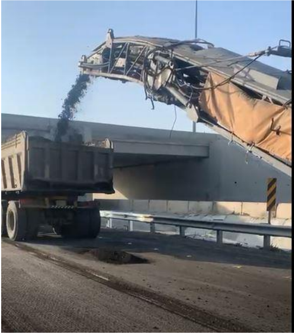
50mm scrapping works
